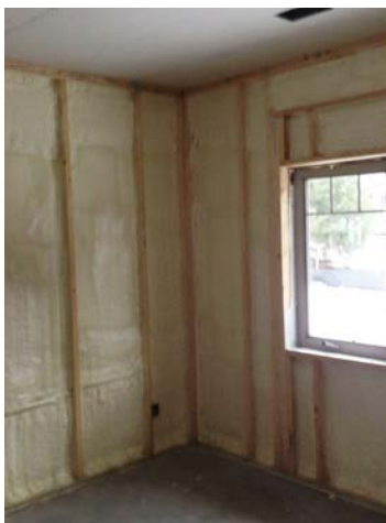
Three inches of closed-cell spray foam provide a low-permeable, air sealing and insulating layer in the wall cavities.
