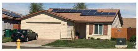
GTI began efforts on a California Energy Commission project to demonstrate the potential of ZNE homes that generate as much energy as they consume. GTI is developing and testing advanced energy efficiency packages using low-cost construction methods, high-performance housing techniques, and solar PV in two identical homes: one all-electric and one mixed fuel. The project is being conducted with Habitat for Humanity in a new affordable housing community in Stockton, California.
